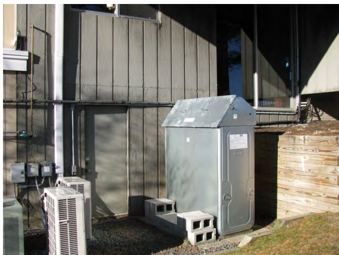
Photo 5 – 275 gallon #2 AST in containment
