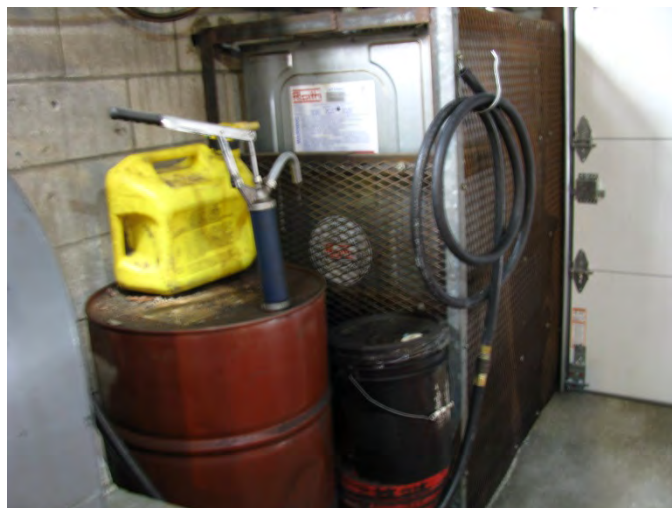
Photo 24 - #2 Fuel oil AST in garage
