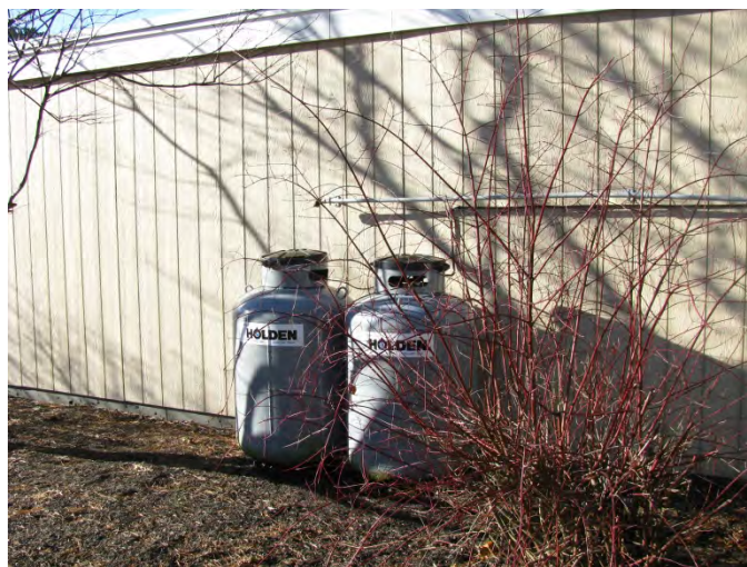
Photo 6 – Propane tanks for kitchen
