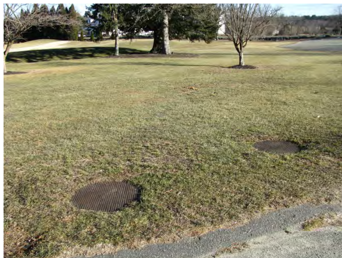
Photo 42 – Septic system manholes
