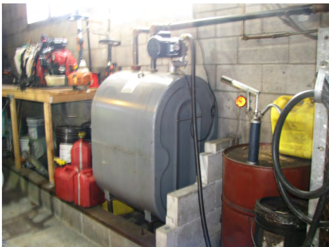
Photo 23 – Diesel fuel AST, lubricating oil drum
