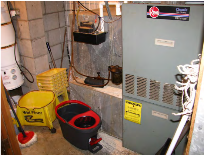
Photo 8 – Clubhouse furnace, overhead feed lines
