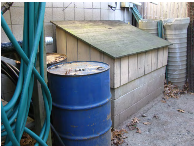
Photo 33 – Containment for waste oil drums
