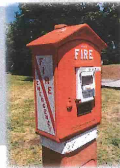
Sigcom Radio Boxes are the ideal replacement for service intensive hardwire connected Master boxes like the one shown here
